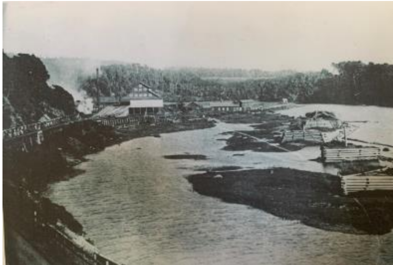
Second mill site, with crib wall structures in estuary.
